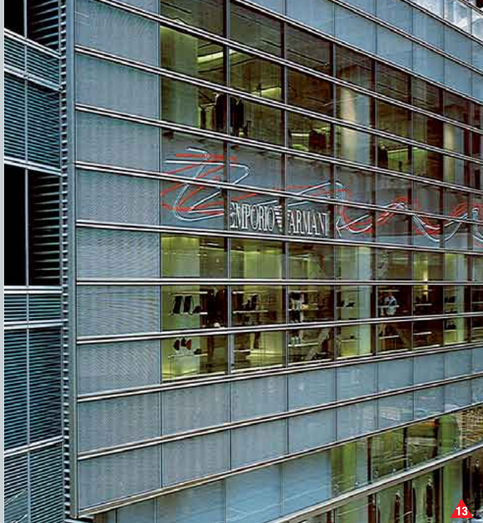
Chater House, Hong Kong, China
